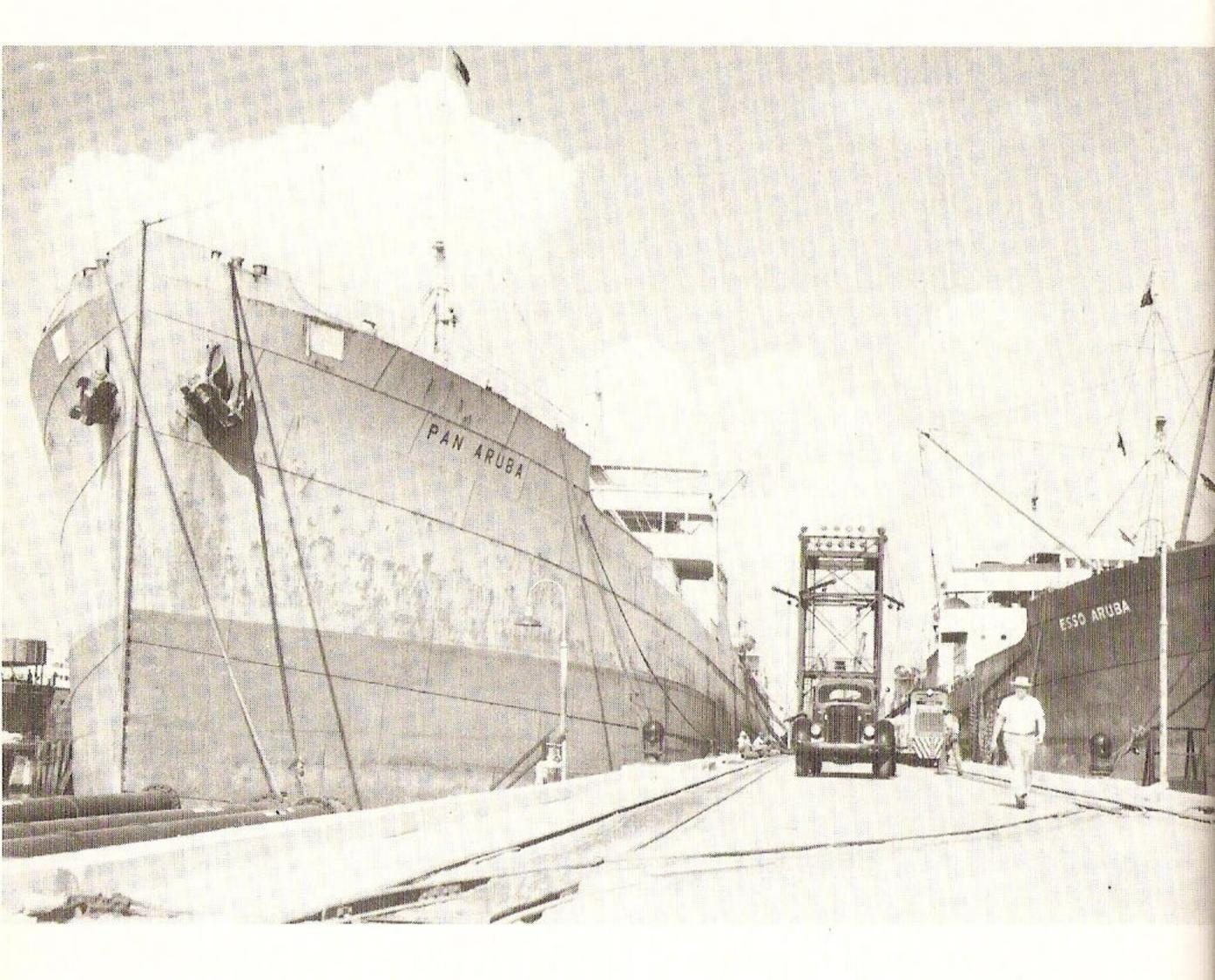
Aruba's own tankers, the **Pan Aruba** and the **Esso Aruba** both at finger pier 1. This rare photograph shows one of the Brookville 10-tonners working along the right side of the pier, probably switching flatcars beneath the cargo crane in the distance. Note the crossover track in the foreground, and the construction of the track, so that it would not interfere with vehicle operation.
