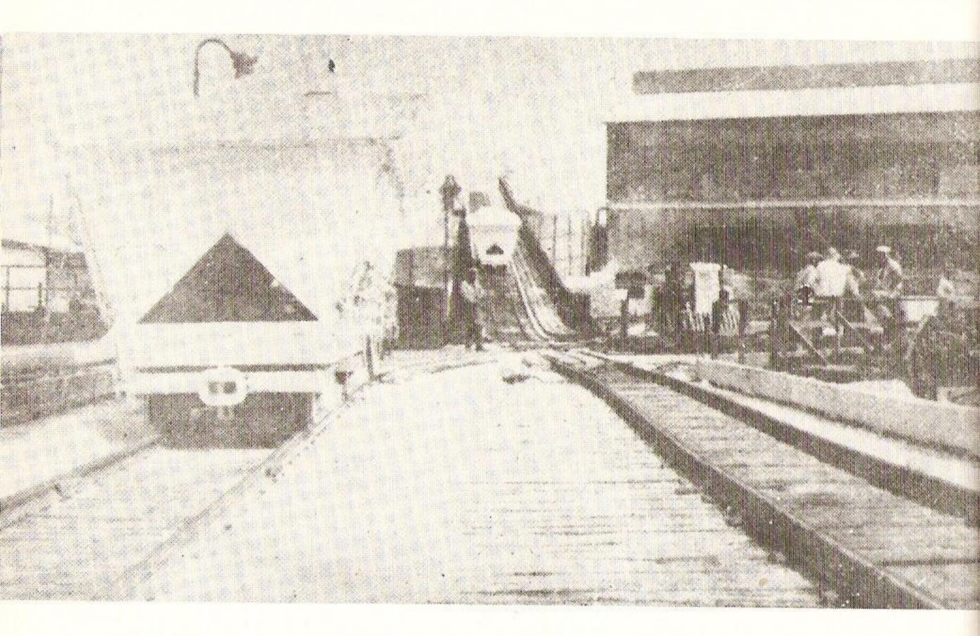
The sulphur storage area was the scene of much railroad activity at Lago. Hopper cars of the yellow mineral were brought from shipside to the acid plant area by locomotives, such as the on in the right distance. Then the cars were winched to the top of the ramp in the center distance, where the sulphur was dumped to await conversion to sulphuric acid.
